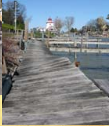
Roller coaster walkway before being fixed
